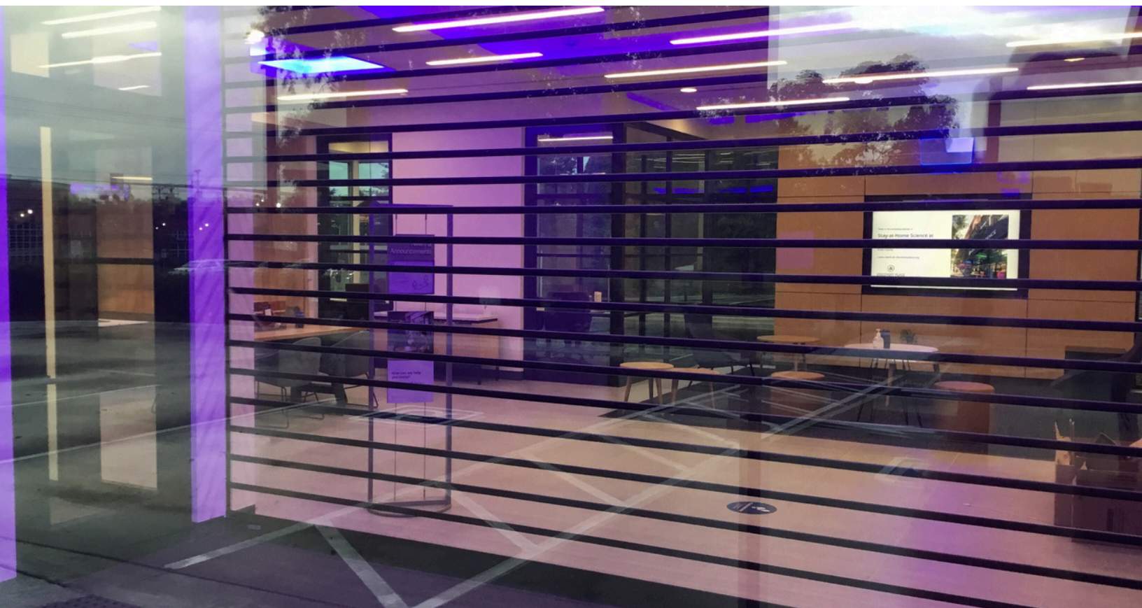
Black anodized TR4 provides striking security complement to this lobby area.
