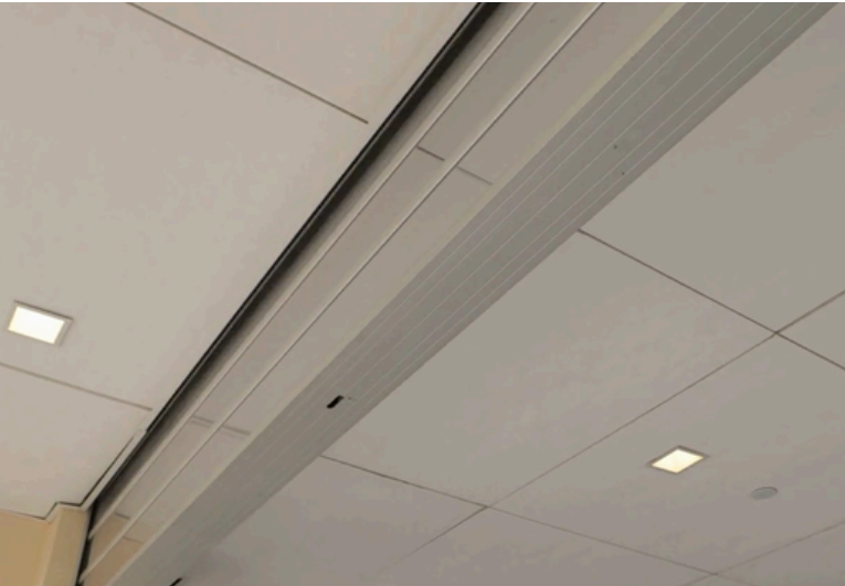
Base slat bottom plate can be tailored to hide ceiling opening when shutter is open.
