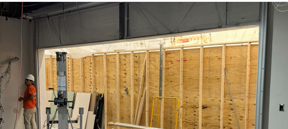
Step 1: XL integrated into pharmacy remodel along with other construction.
