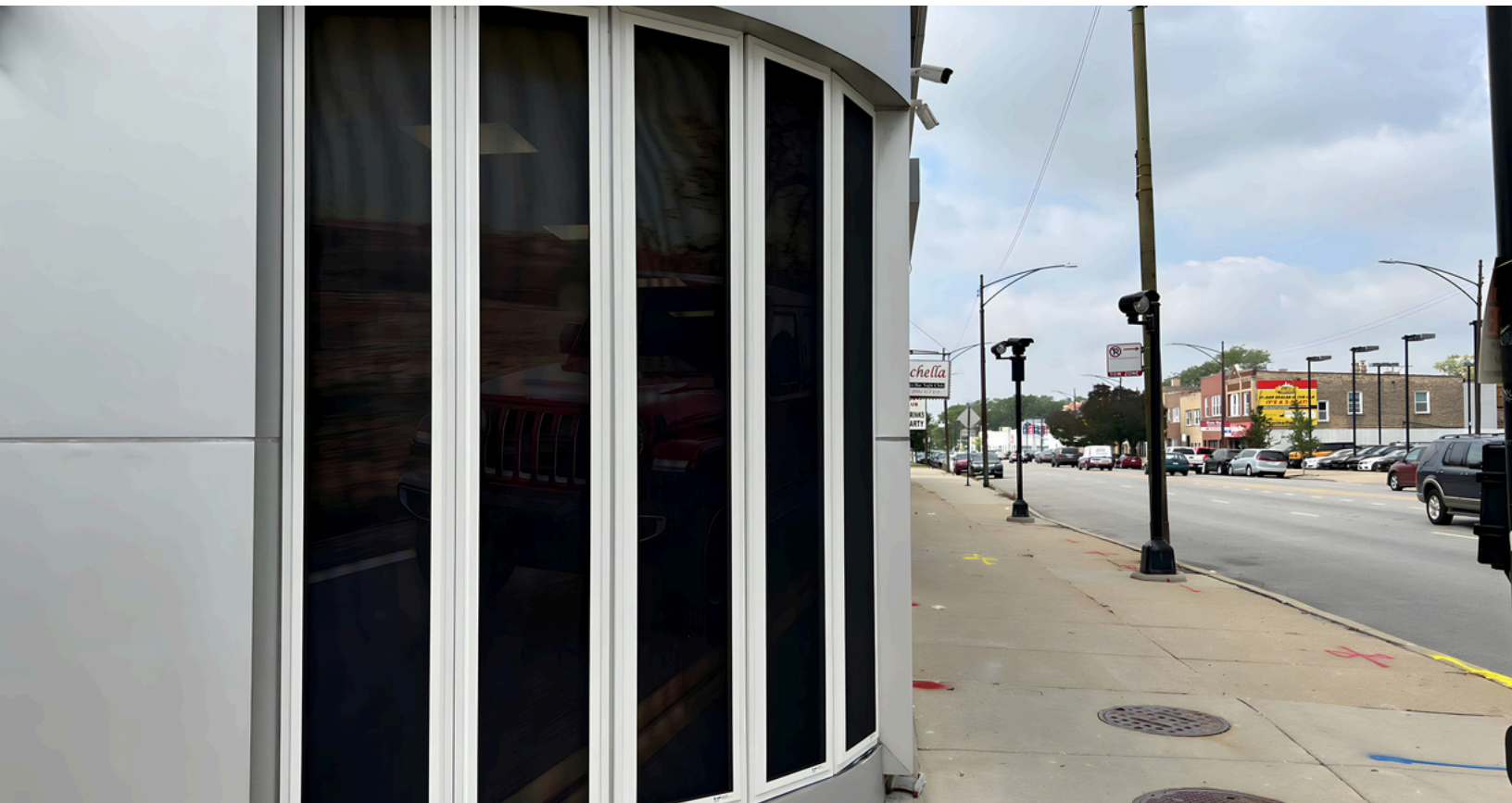
Fixed screens secure multi-pane, curved, sidewalk-adjacent windows at a California business.
