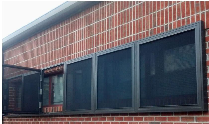
Egress screens installed on back, ground level windows per code.
