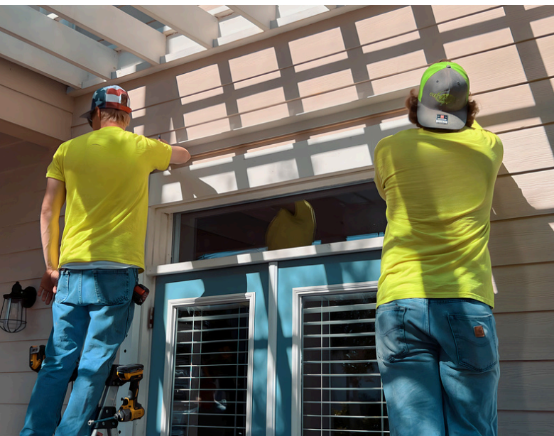
Expert QMi dealer partners preparing another exterior Qcompact shutter over the home's double door.
