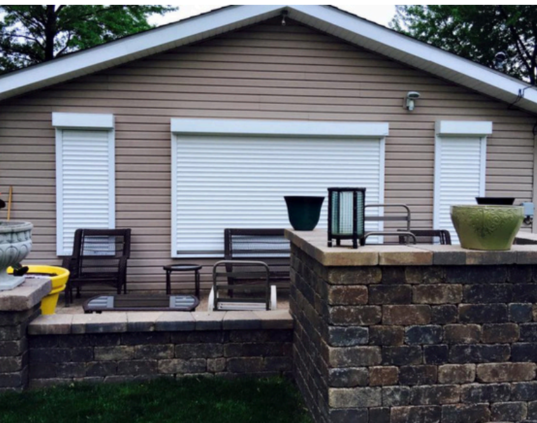
Exterior mounted Qcompact shutters were installed over various openings to bolster the security of the home's rear.
