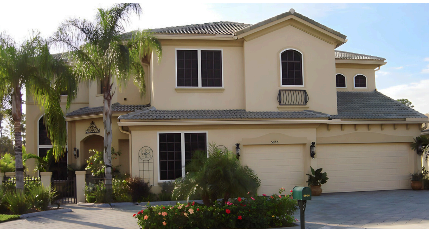
Rectangular and shaped screens secure a Florida home from hurricanes and potential intruders.
