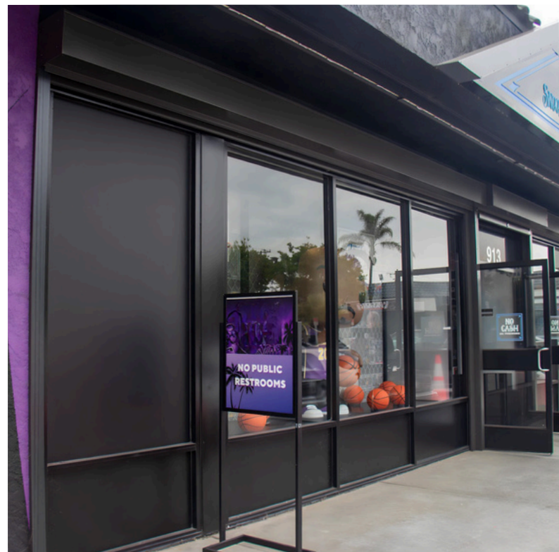
An exterior mounted AL8 shutter seamlessly blends in with the storefront entrance and goes unnoticed during operating hours.
